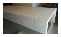
The wooden frames on the towers worked as a stand to do the painting and mortar joint work. Once on the stage, the top frame was removed and the tower stood on the bottom support.
