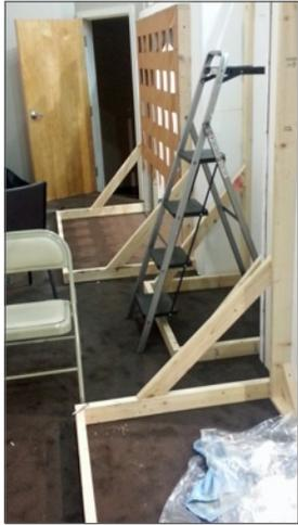
Once the four sections were butted together on stage, the base frames were attached to the two shorter sections. We made use of duct tape and 3 inch nails inserted at opposing angles thru the adjoining panels to hold them all together in a manner where they could be taken back apart with minimal damage.
